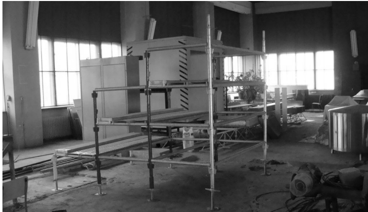
Fig. 3. Back view of temporary steel grandstand considered in the study
